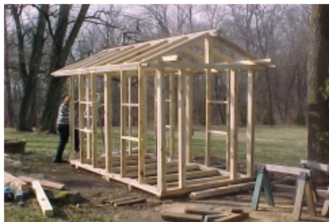
Figure 10.—The nearly completed frame.
