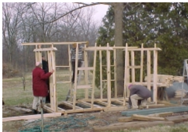
Figure 9.—In progress assembly of the frame.
