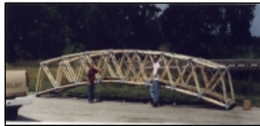
Figure 5.—A 35-ft LPSA bridge built from five-year-old SDT.
