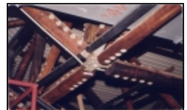
Figure 2.—The Minnetonka SDT joint.
