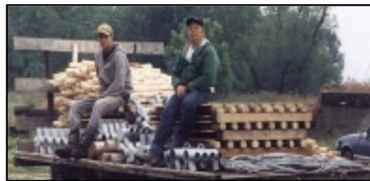
Figure 6.—All bridge parts fit on a small trailer.
