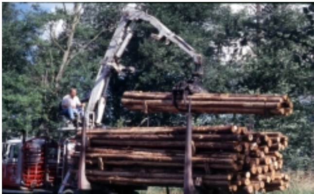
Figure 5.—Stream habitat and bioengineering logs constructed from smallwood are unloaded at a project site near Enumclaw, WA.
