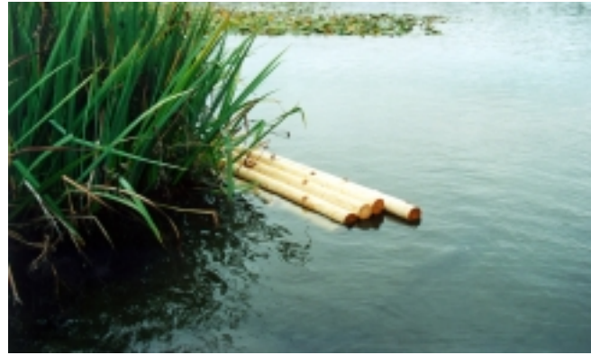
Figure 6.—Floating raft with elliptical surface was constructed from untreated pole stock to provide basking habitat for turtles, amphibians and birds in a pond.
