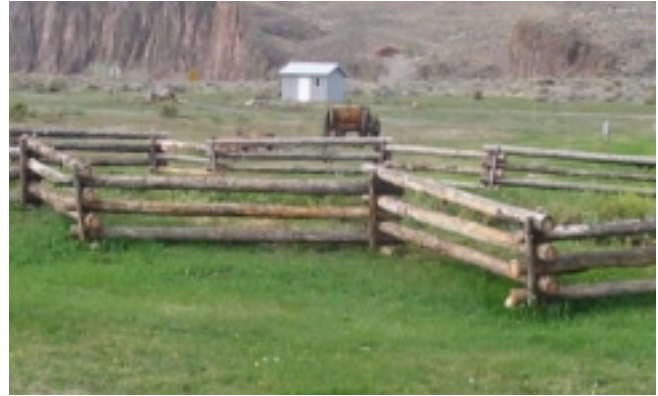
Figure 2.—Virginia stacked rail fence near Salmon, ID, provides safety barrier along creek in a park setting.
